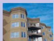
The Ridge at Hermitage - 126 units
