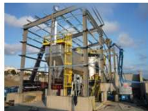
Dockside Green technology
