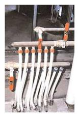
Uponor manifolds supply hot and cold water to fixtures in over 300 units of a residential high rise.
