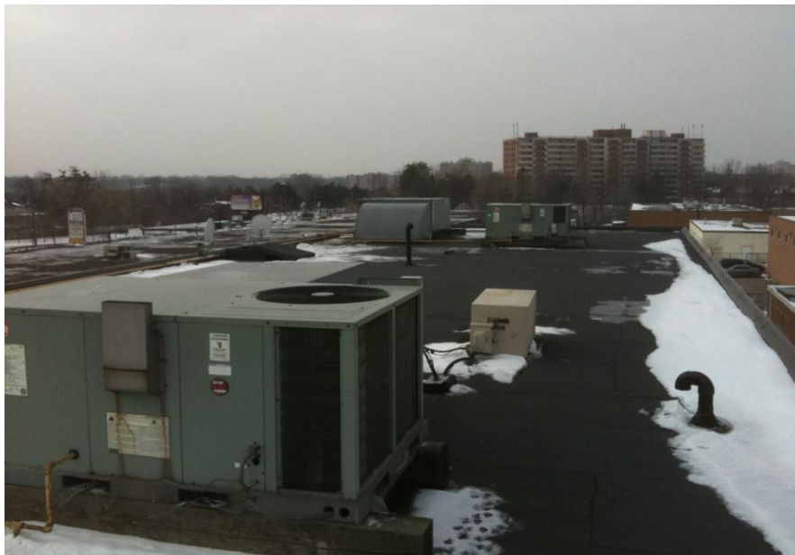
Photo #6: 3 Building Heating & Cooling Units at Roof
