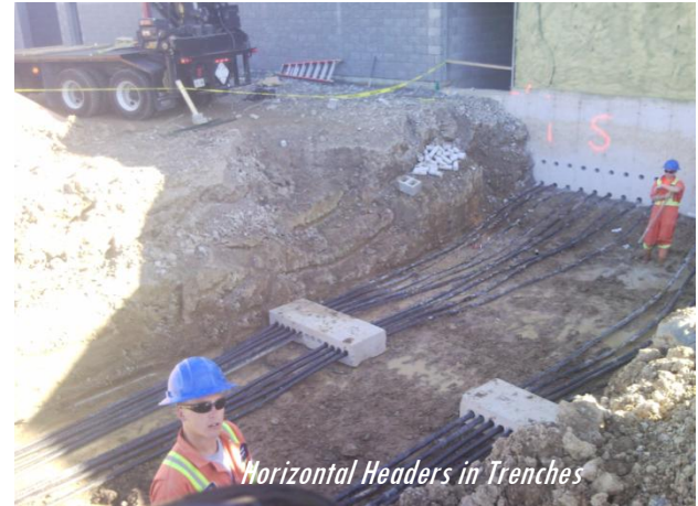
Horizontal Headers Connected to 3/4" HDPE Pipes
