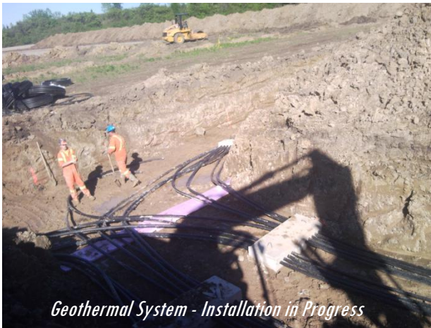
Horizontal Headers Connected to 3/4" HDPE Pipes
