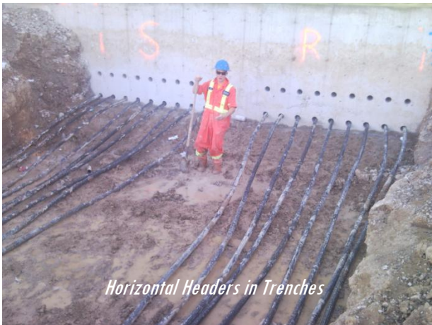
Geothermal System - Installation in Progress
